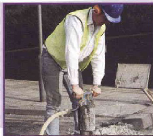
5 The workman mends our roads.
